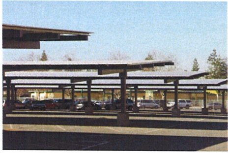
1A CARPORT MOUNTED PV SYSTEM NTS
