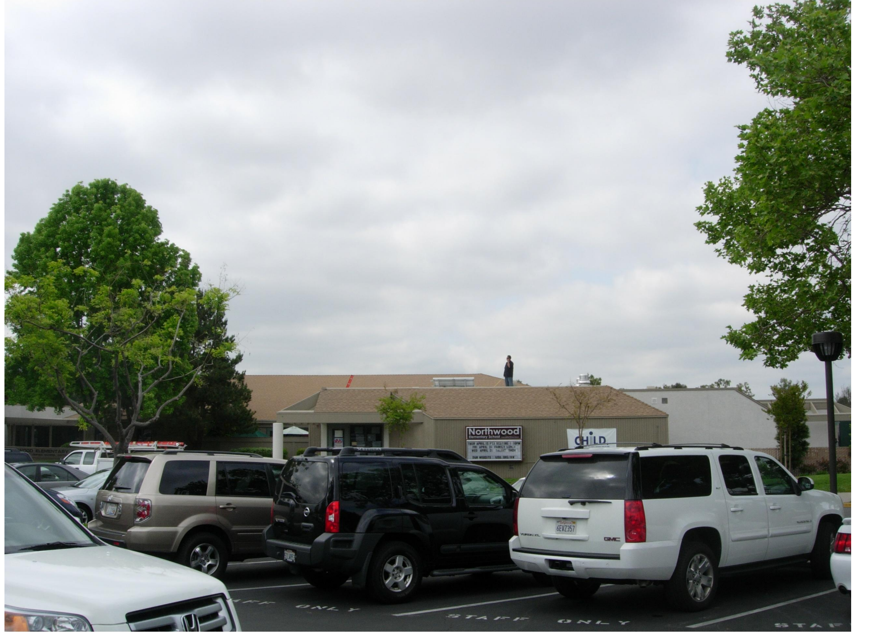
1 F1 NTS PHOTO FRONT OF BUILDING
