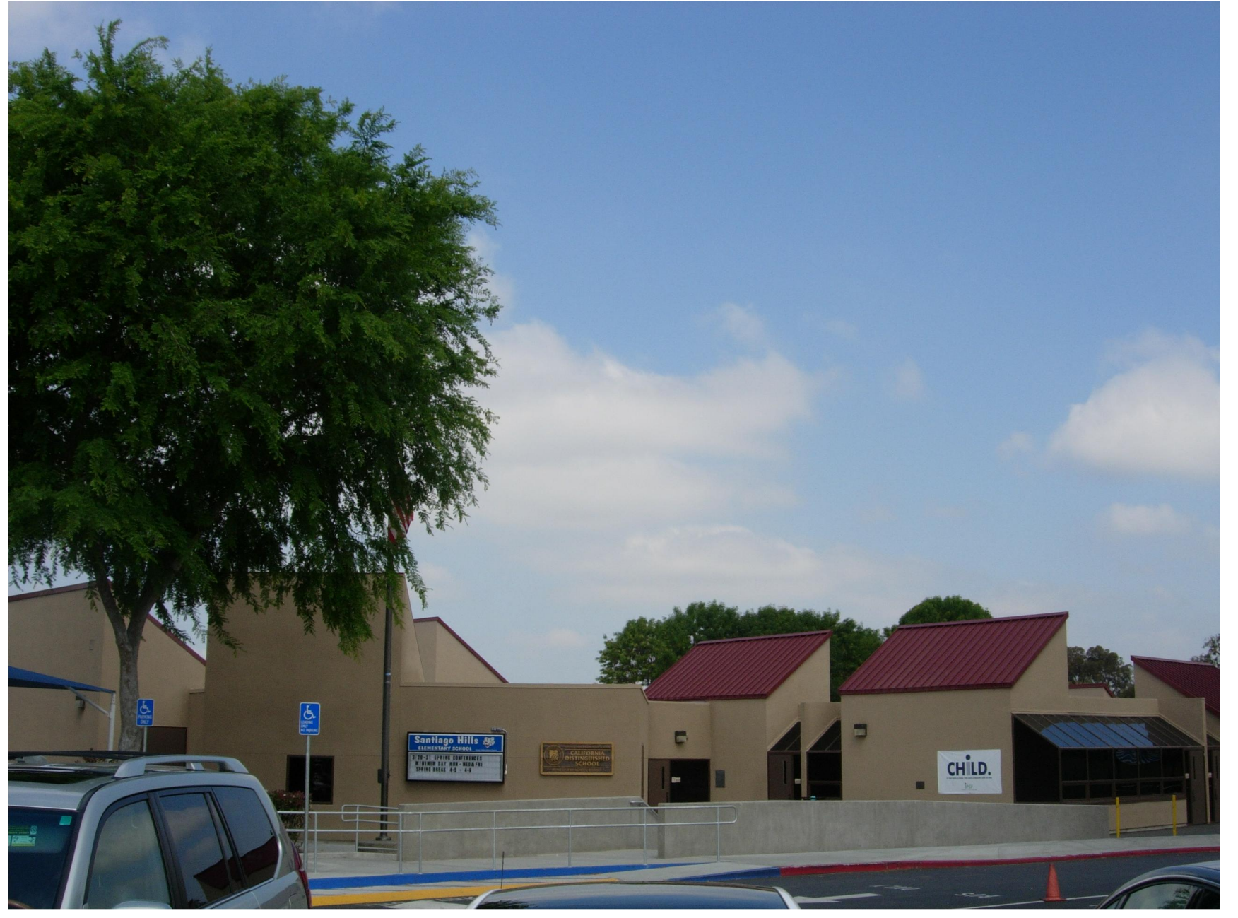
1 F1 NTS PHOTO FRONT OF BUILDING
