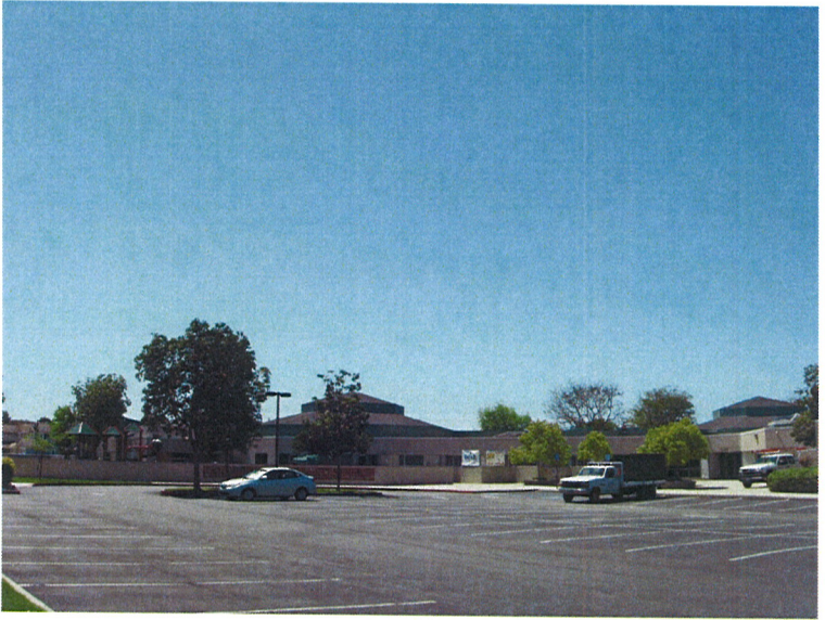
1 F1 NTS PHOTO FRONT OF BUILDING
