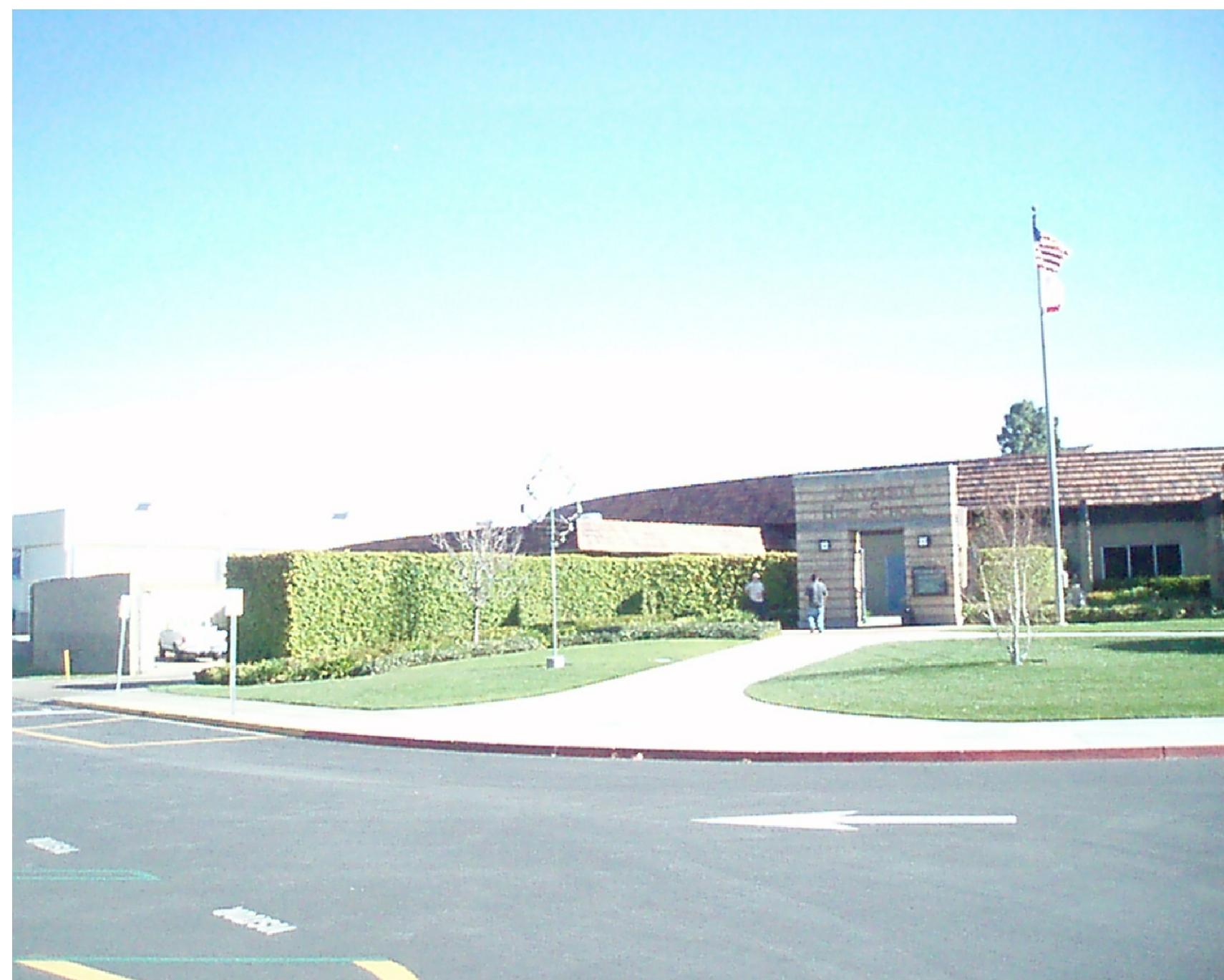
1 F1 NTS PHOTO FRONT OF BUILDING "A"
