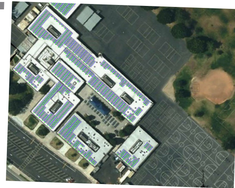
An aerial view of the proposed solar installation at Rancho San Joaquin Middle School. Under a "mega" power purchase agreement, the district went from experimenting with installing one solar panel on one school to full rooftop installations on 18 schools.
